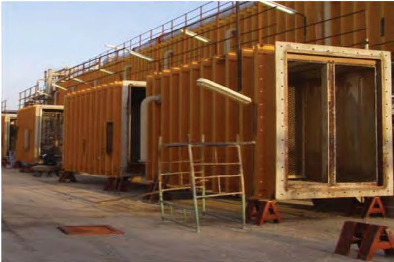
Process optimization of two 1800 m 3 /day MED-TVC Units – Lavan Island, Lavan Oil refinery Co.
