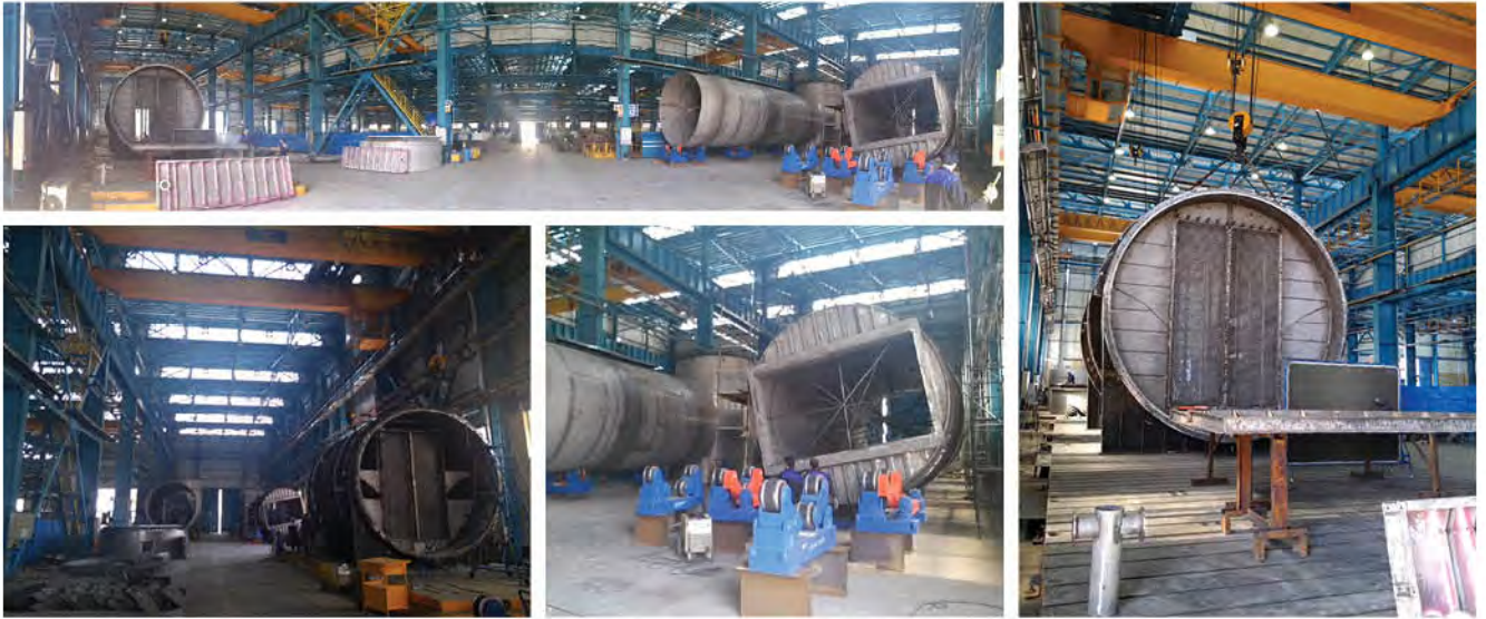
Complete Design of four 4500 m 3 /day MED-TVC Unit – Qeshm Island, Qeshm Water and Power Co.
