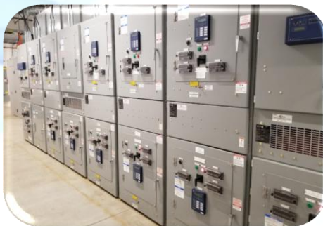
MV Switchgears
